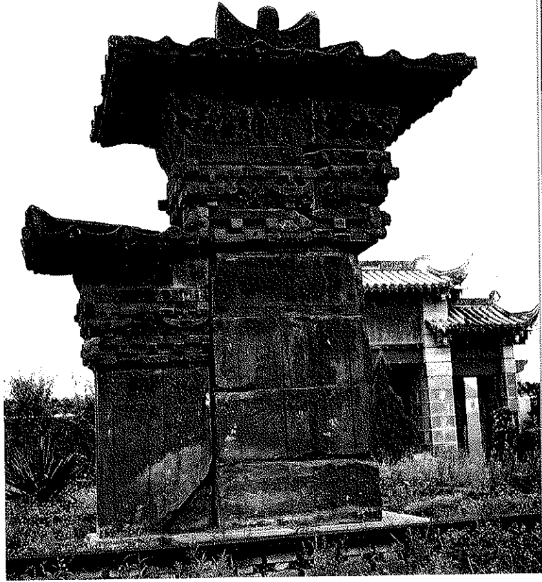
Figure 2.22. Double-body gate tower from the tomb of Gao Yi in Ya'an county, Sichuan province
