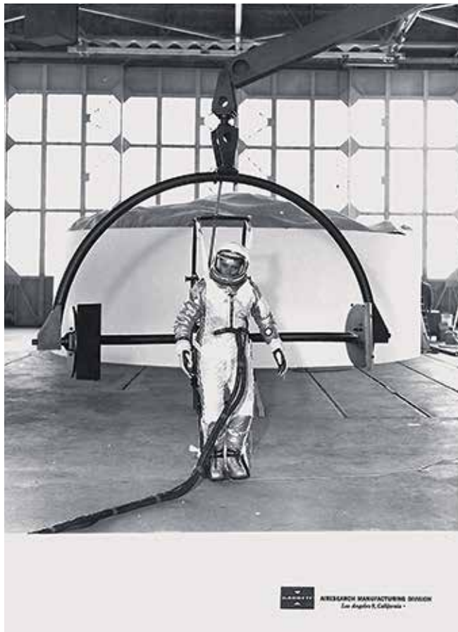
⑤ Engineer testing astronaut's self-locomotive capabilities in lunar gravity simulation device, ca. 1967
